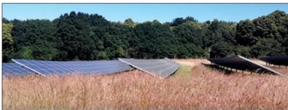
Figure 6: Sites where a “Shade Cut” has been employed during the growing season to prevent shading of panels, but allow flowering meadow elsewhere
